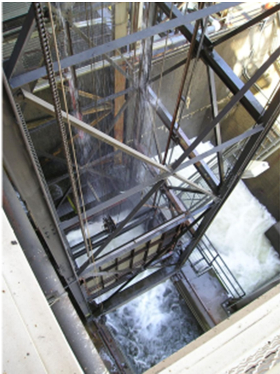
Fig. 4 The Robert E. Garrett fish lift (elevator) at the Holyoke Dam on the Connecticut River, USA. Photo credit: City of Holyoke
